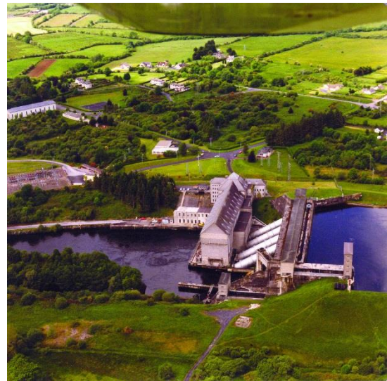
Hydro-Power Station at Ardnacrusha (The Shannon Scheme)
