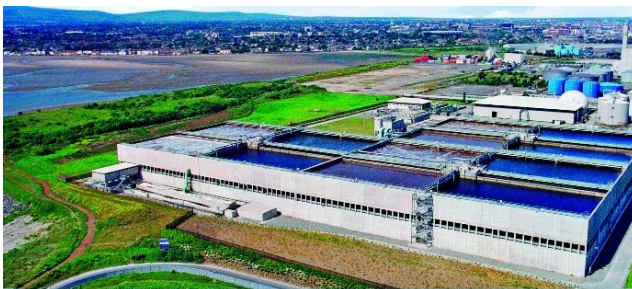
Ringsend wastewater treatment works, Dublin
