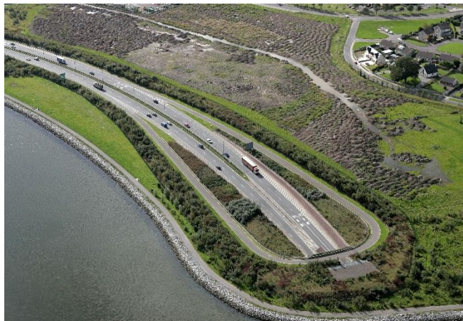
Southern approach to river Lee road tunnel
