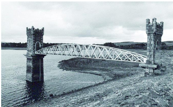
The Vartry reservoir, county Wicklow
