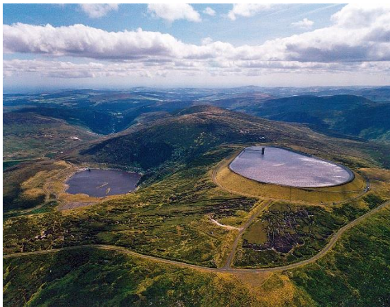
Turlough Hill Pumped-Storage, county Wicklow
