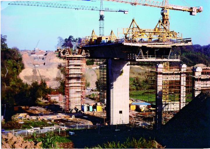
Construction of West Link Bridge on M50
