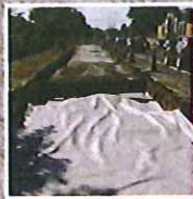
Fibertex F-2B Separation function N6 Ballinasloe, Galway County Council
