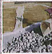
Fibertex F-4M Separation and Filtration Functions Equestrian Arena, McKee Barracks, Dublin
