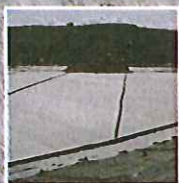
Fibertex F-1200M Protection Function Ballealy Landfill Site, Fingal County Council
